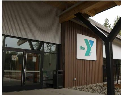
from our Eternal Collection. With its unique depth and dynamic light interaction, Ironstone provides a warm, contemporary color that complements wood and concrete materials and contrasts other metal elements. Its robust FEVE coating is a building manager's dream, with outstanding durability, graffiti resistance, and low long-term maintenance requirements.
