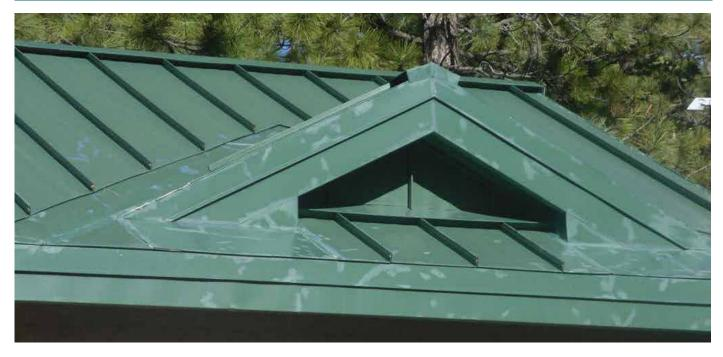
Scratches and very minor damage may occur during handling and installation of painted roofing and wall panels. In these instances, it may be desirable to use touch-up paint to repair the blemishes. Keep in mind, touch-up paints are quick fixes and when used properly, will result in a satisfactory appearance. Misuse or over-use can result in spoiling the overall appearance.
